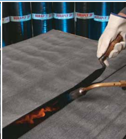
B - Welding lap joints
